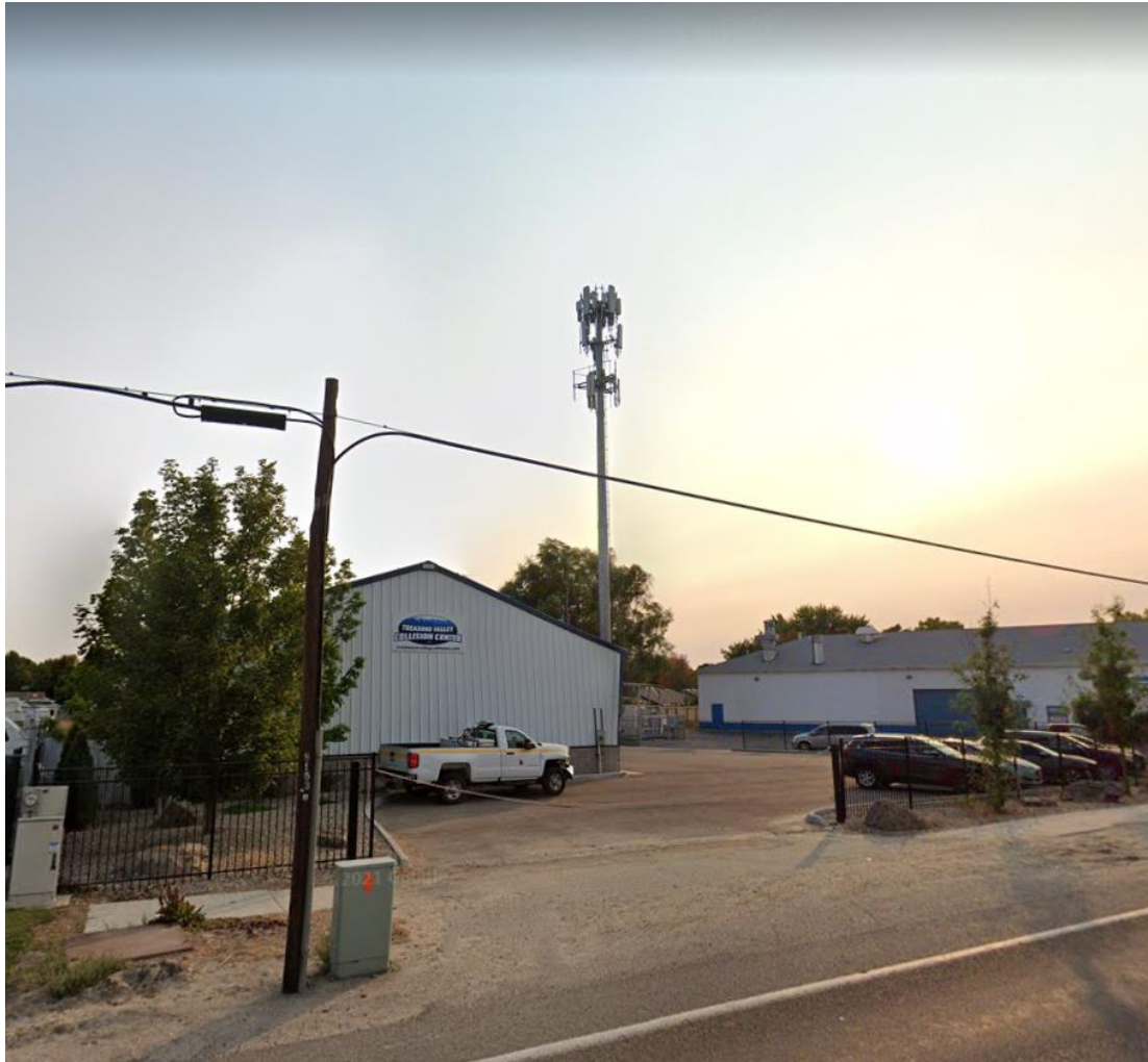
SUBECT TOWER LOOKING SOUTHWEST FROM W. STATE ST.
