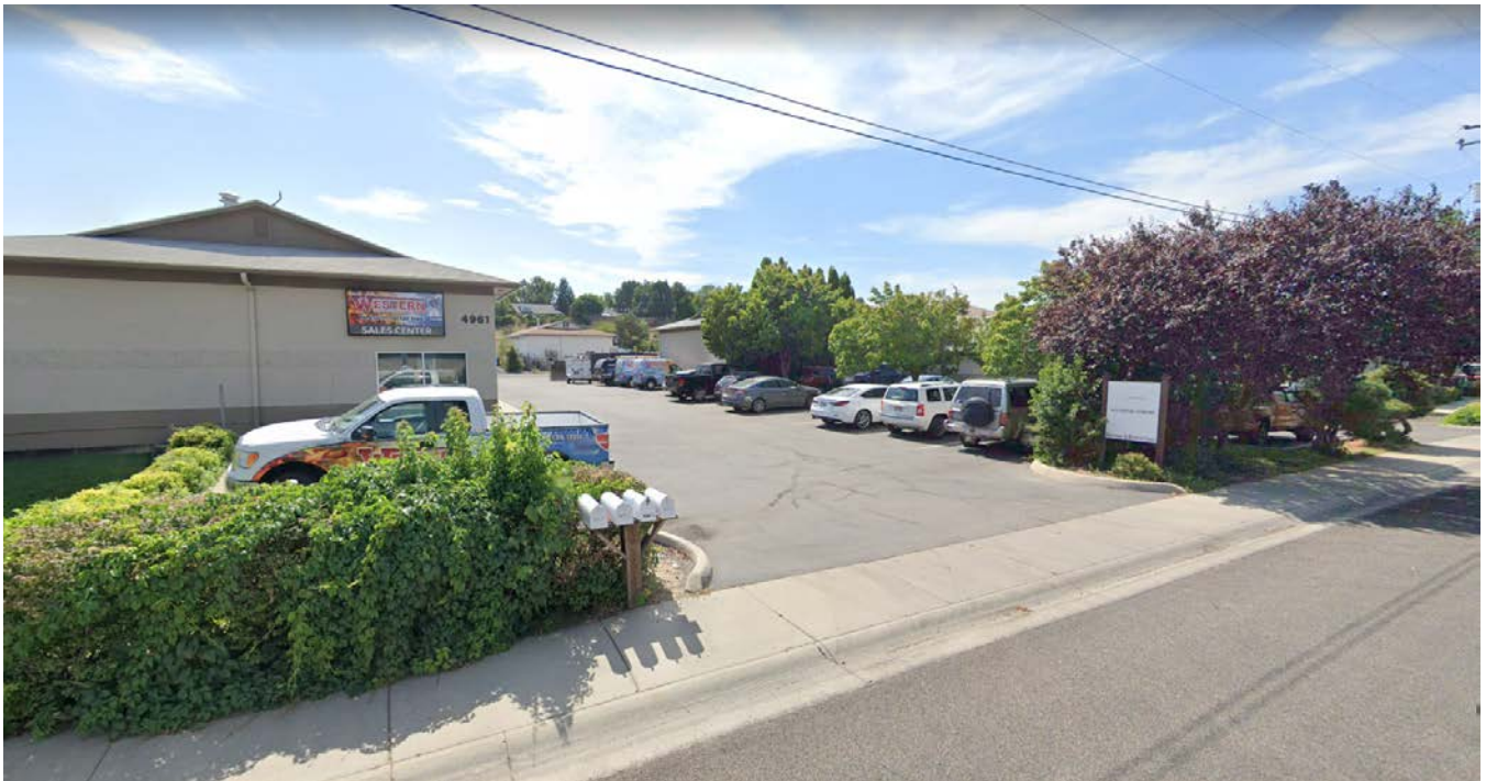
Figure 3: Western Heating and Air Sales Office (Google Streetview, 2019)
