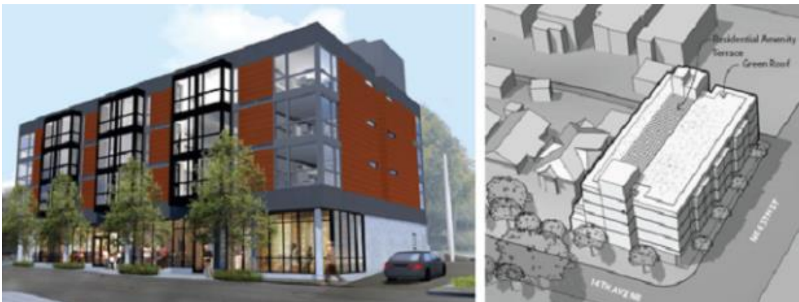
Studio apartments over ground level retail in Seattle's Roosevelt neighborhood (images courtesy of Weinstein A+U).
