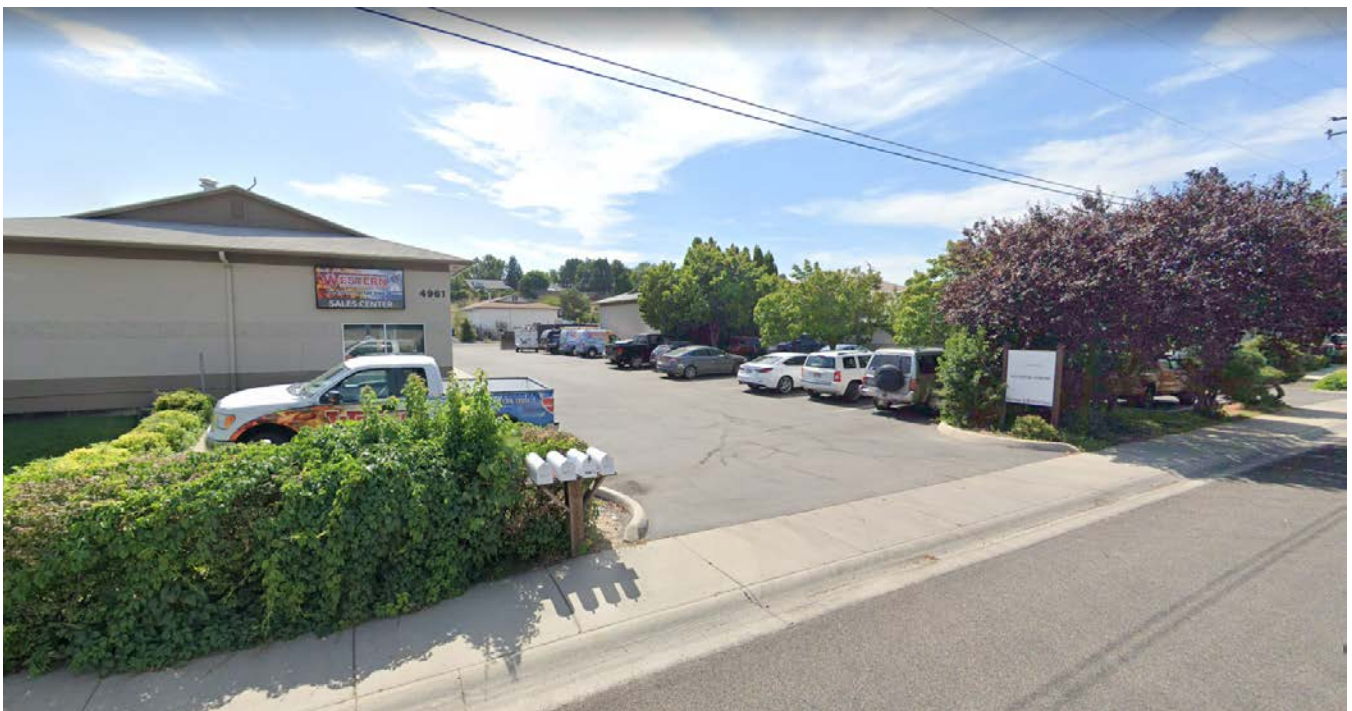
Figure 4: Western Heating and Air Sales Office without Certificate of Occupancy (Google Streetview, 2019)
