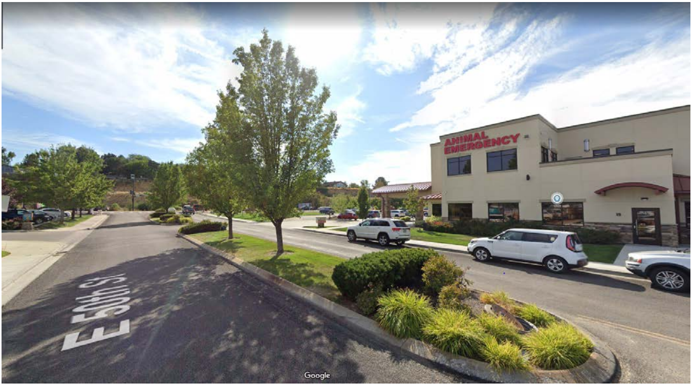
Figure 5: Existing site conditions along 50th Street
